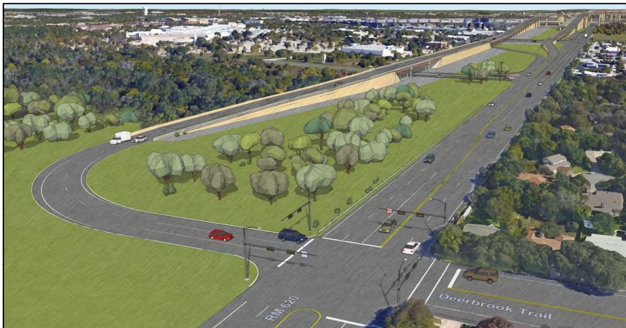
Figure 8. Build Alternative: Artist rendering (birds-eye view) of new button-hook exit from northbound US 183 direct connector ramp to RM 620 west.
